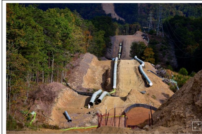
FILE PHOTO: Lengths of pipe wait to be laid in the ground along the under-construction Mountain Valley Pipeline near Elliston, Virginia, U.S. September 29, 2019. Picture taken September 29, 2019. REUTERS/Charles Mostoller
